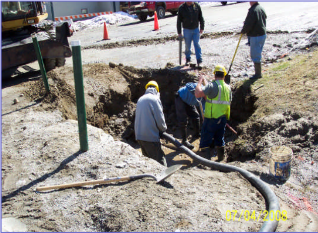
Gurney Brothers Construction repairing water line infrastructure
